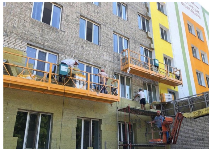
Restoration of the city hospital in Trostianets, the Sumy region
